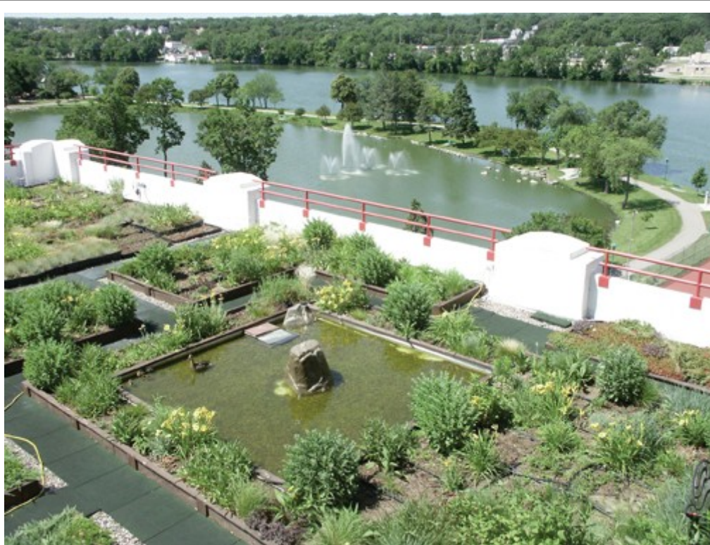
Figure 6–8: Green Roof at ABC Supply Company, Inc.
