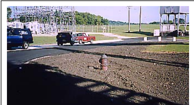
Figure 6-5: "Before" grass growing on We Energies' landscaping with Scott's 10% bottom ash topsoil blend at We Energies' Milwaukee County Power Plant.
