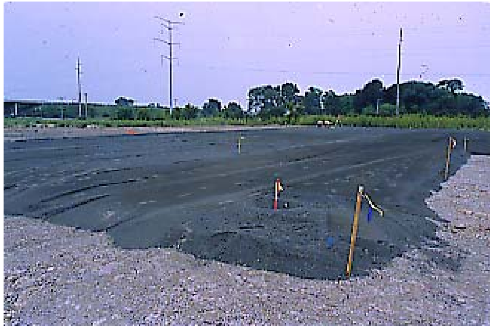
Figure 6-3: Bottom ash base course for concrete building slab in Racine, Wisconsin
